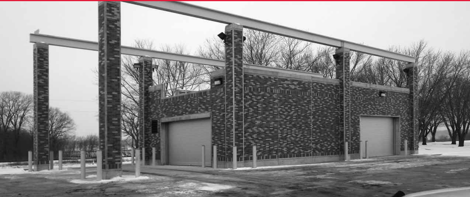
Trinity Fabricators was awarded the contract with the Army Corps of Engineers for the Flood Control Building at Lock and Dam #20 in Canton, Missouri.
